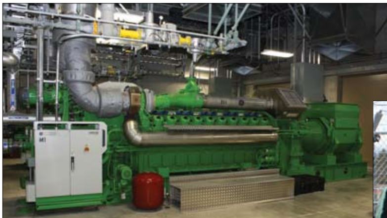
One of the two 3-megawatt Jenbacher natural gas engines that power the High Sierra Cogeneration Power Plant.
